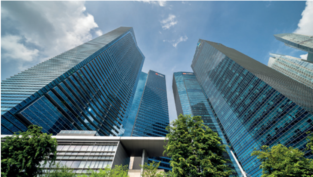
Keppel REIT's sterling portfolio of properties in Singapore includes Marina Bay Financial Centre, an integrated development comprising three premium Grade A office towers and the subterranean Marina Bay Link Mall.
