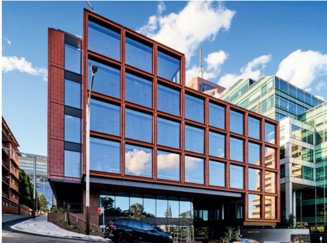
2 Blue Street achieved practical completion in April 2023 and has attracted strong interest from potential tenants.
