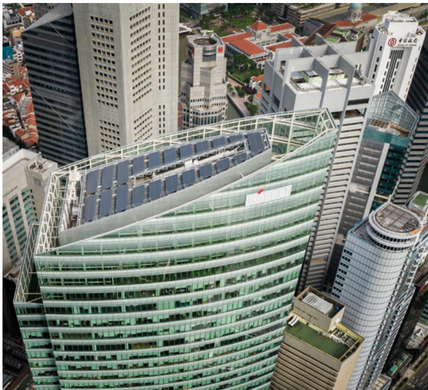
The Manager taps on renewable energy and implements energy optimisation initiatives across its portfolio. Pictured are the solar panels atop Ocean Financial Centre.
