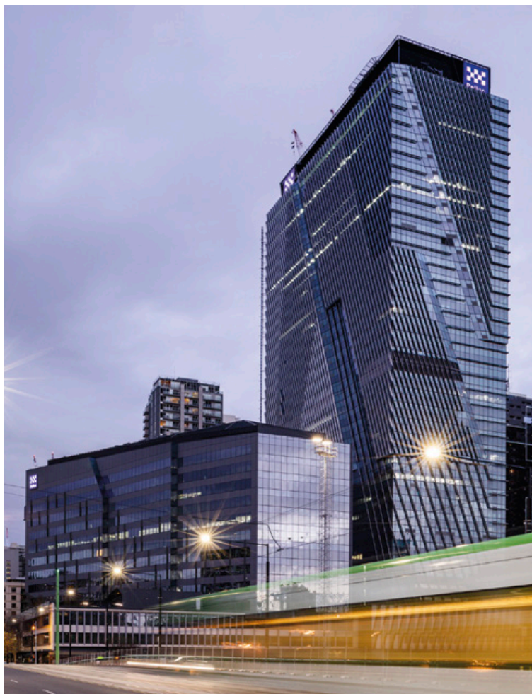
In Melbourne, Victoria Police Centre achieved practical completion on 9 July 2020 and serves as the headquarters for the Victoria Police.
