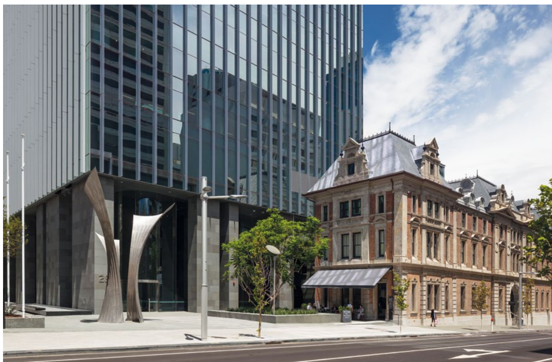
David Malcolm Justice Centre is located in Perth's CBD and has the Minister for Works – Government of Western Australia as its principal tenant.
