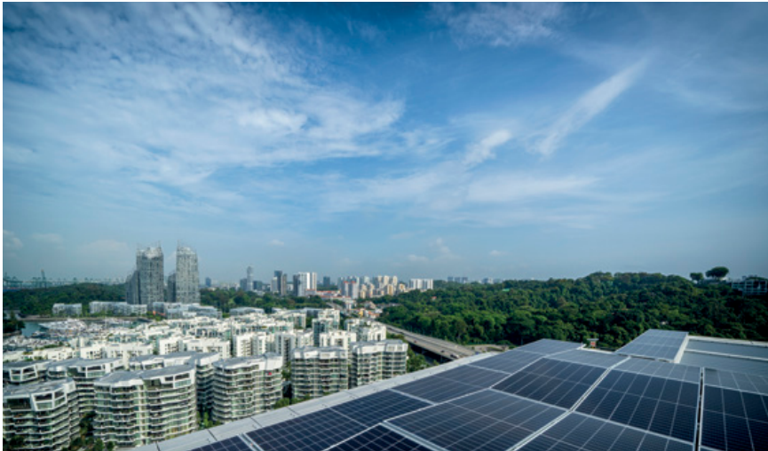
◀ Keppel Bay Tower is Singapore's first commercial development to be fully powered by renewable energy. Its green features include on-site solar panels (pictured).
