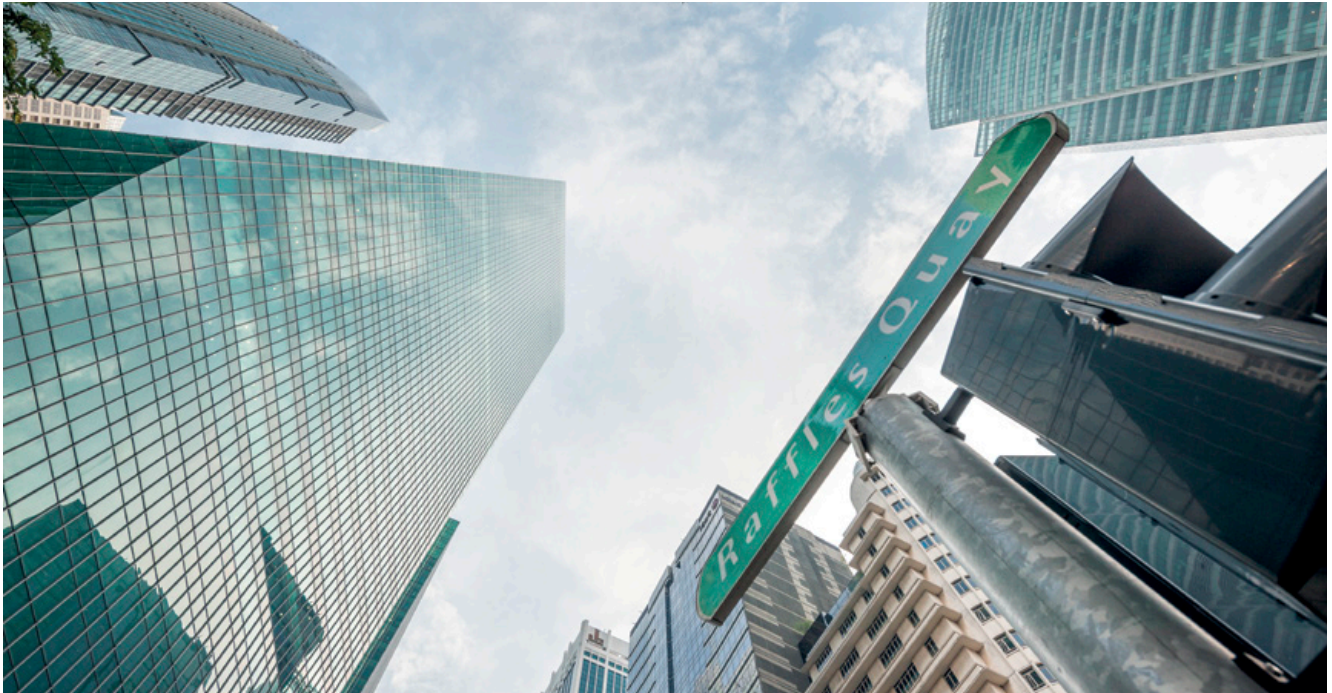
Keppel REIT's Grade A commercial portfolio includes One Raffles Quay (pictured), a landmark commercial development in Singapore's CBD.
