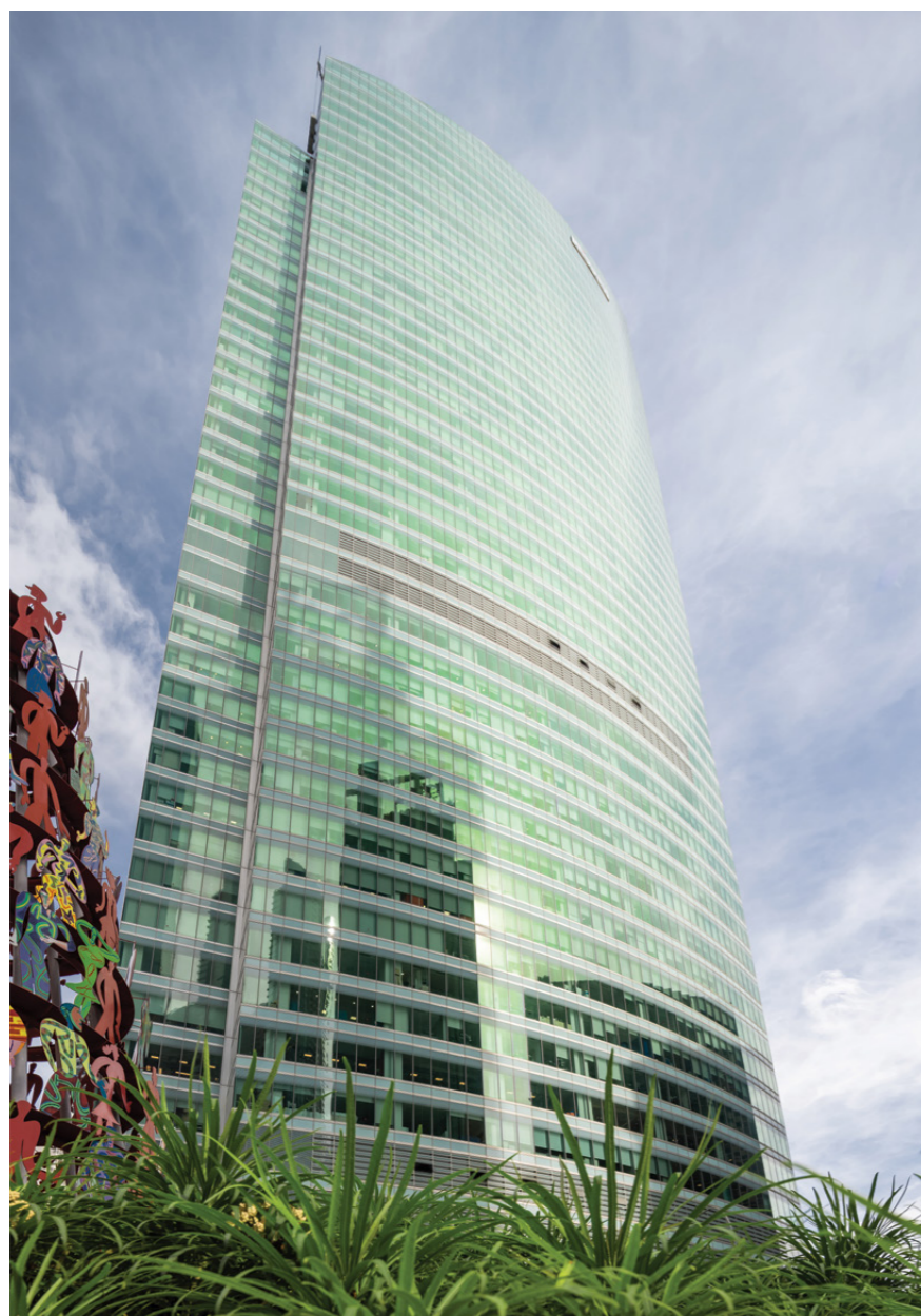
Ocean Financial Centre – Singapore's first commercial building to achieve WELL Health-Safety Rating by the International WELL Building Institute, for its robust health and safety management.
