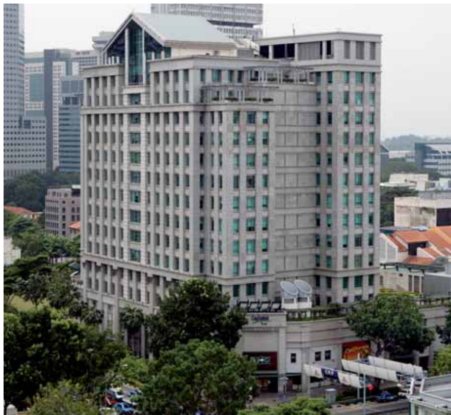
Bugis Junction Towers is part of an award-winning integrated mixed-use development.
