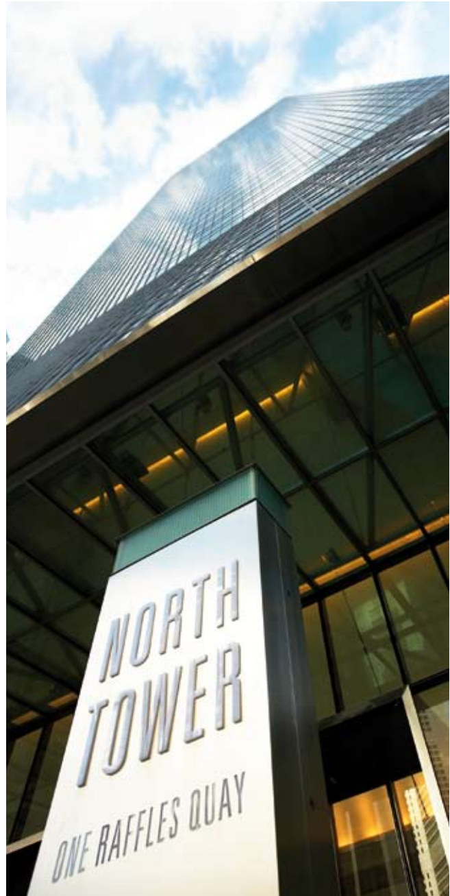
One Raffles Quay is one of the newest, state-of-the-art buildings in the Marina Bay area
