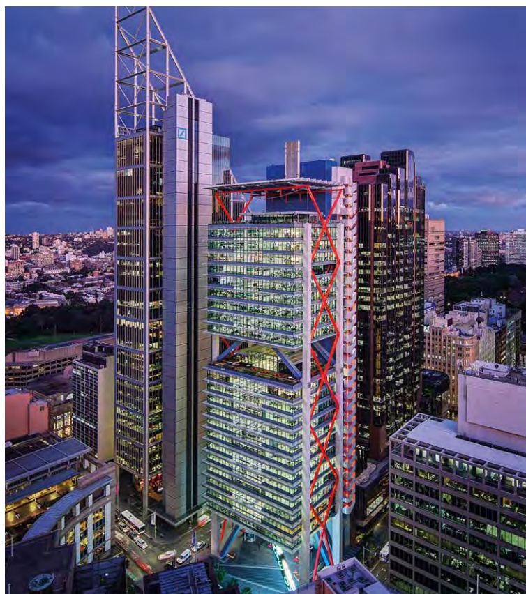
Keppel REIT holds a 50% interest in 8 Chifley Square, a premium grade office building in the heart of Sydney's CBD.
