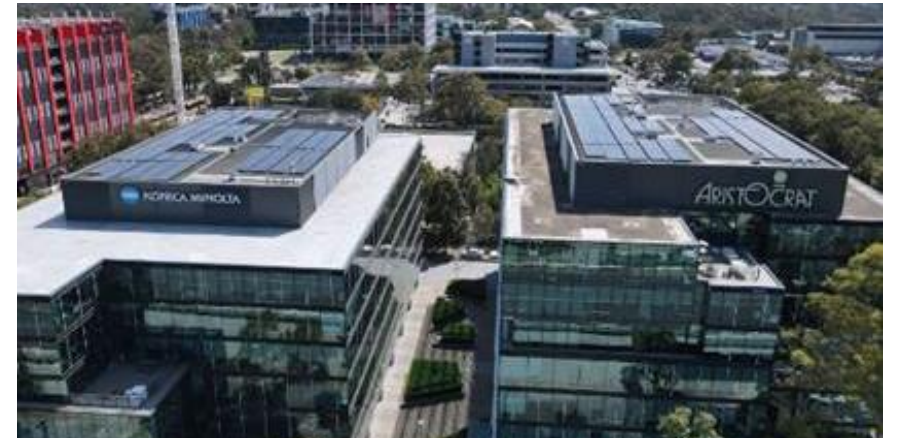
Solar panels were installed at Pinnacle Office Park in Dec 2021 to tap on renewable energy
