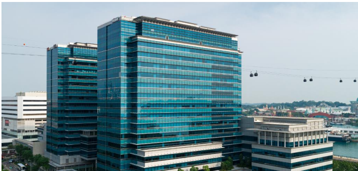
Keppel Bay Tower is Singapore's first commercial building to be certified BCA Green Mark Platinum Zero Energy
