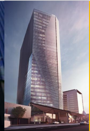
311 Spencer Street Melbourne (50% interest) -Under construction-
