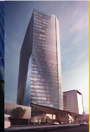
311 Spencer Street Melbourne (50% interest) -Under construction-
