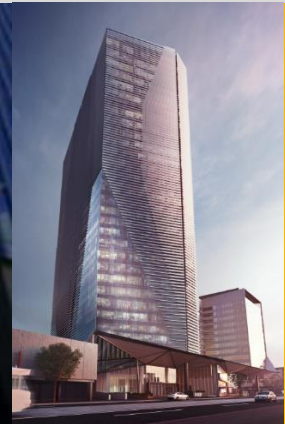
311 Spencer Street, Melbourne (50% interest) -Under construction-
