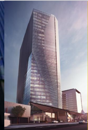
311 Spencer Street, Melbourne (50% interest) -Under construction-
