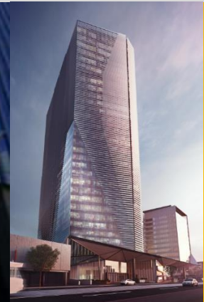
311 Spencer Street Melbourne (50% interest) -Under construction-
