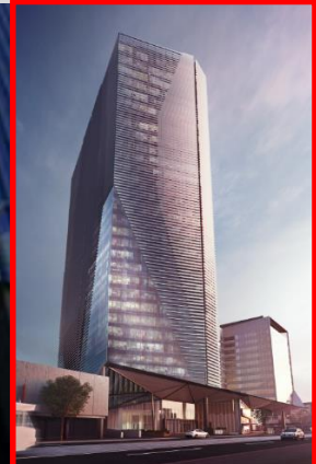
311 Spencer Street Melbourne (50% interest) -Under construction-
