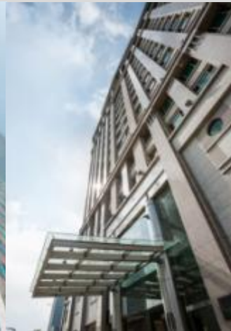
Bugis Junction Towers (100% interest)
