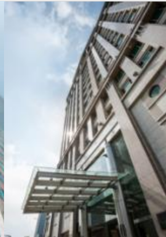
Bugis Junction Towers (100% interest)
