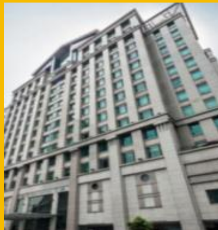
Bugis Junction Towers (100% interest)
