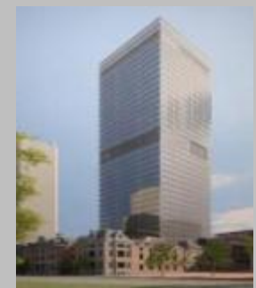
Old Treasury Building Office Tower, Perth (50% interest)
