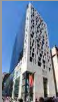
77 King Street Office Tower, Sydney
