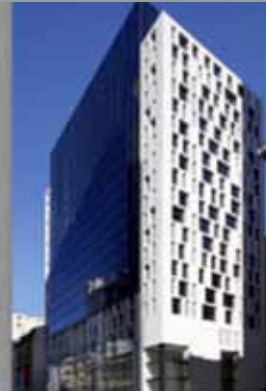
77 King Street Office Tower, Sydney
